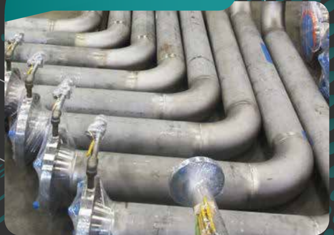
PIPE SPOOL PT TEST
