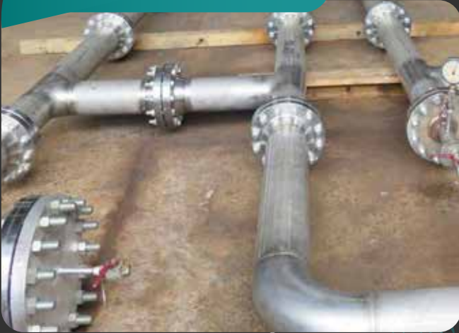
HYDRO TEST SPOOLS
